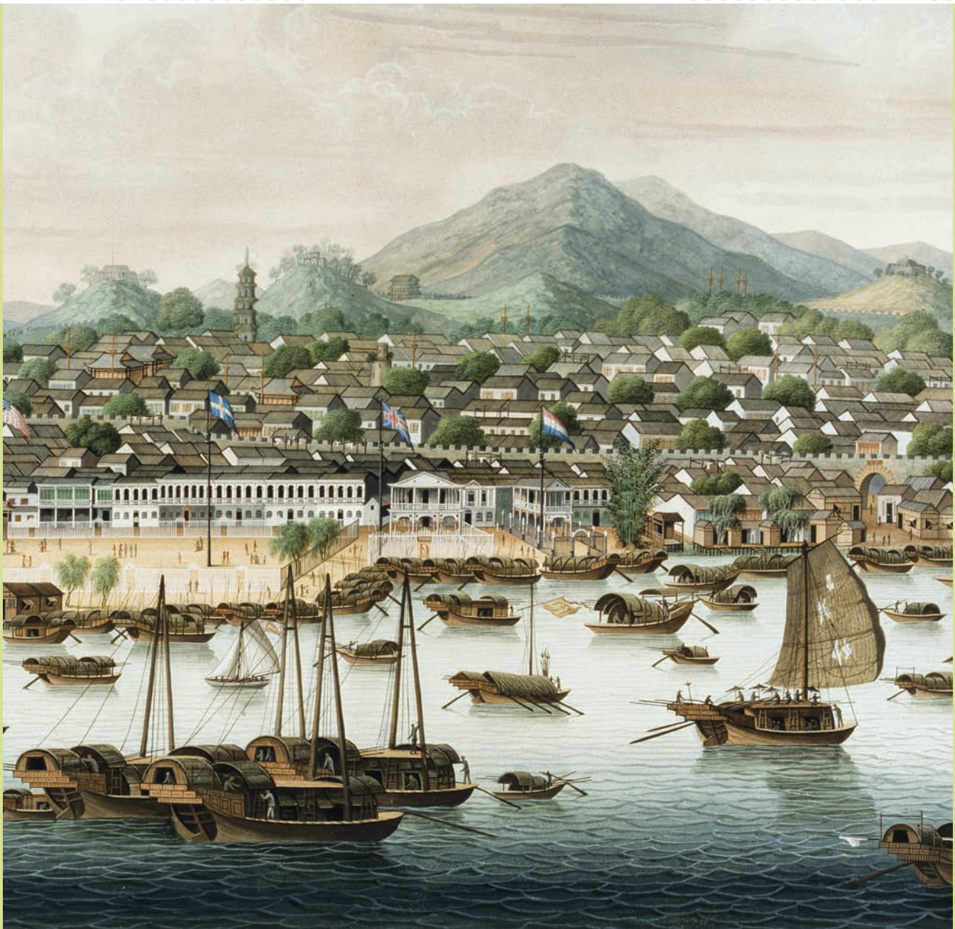
European-style buildings on the waterfront in eighteenth-century Guangzhou, where foreign merchants conducted their business.
